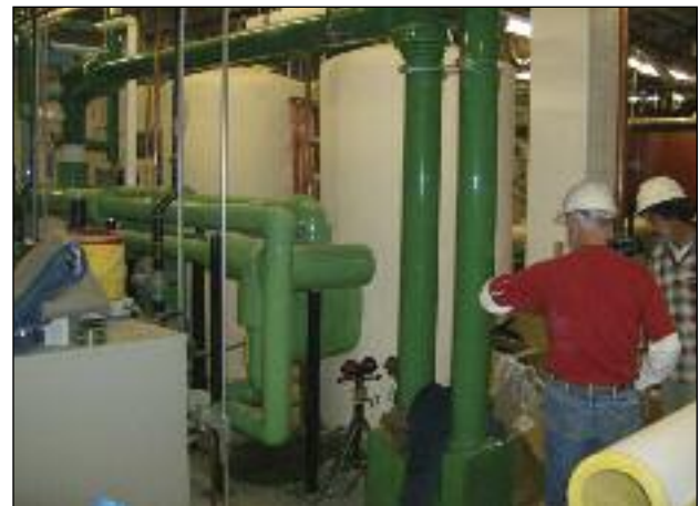
Rainwater storage at the Western Virginia Regional Jail is stored in four 30,000-gallon belowground fiberglass storage tanks. Storage tank selection can be tailored to the site.
