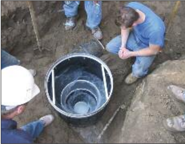
A high capacity vortex filter in action during construction of the Burton School. This pre-tank filter diverts the “first flush” and prevents debris from entering the tank. A single filter can treat roof areas up to 33,000 square feet. (Photo courtesy of Paula Leatherman.)
