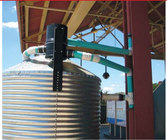
A Wisy vortex filter reduces particulate to 280 microns and is designed to handle the proper gallon per minute flow.
