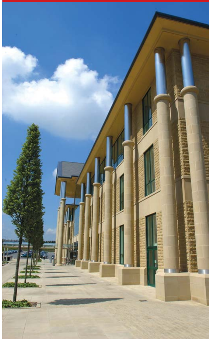
Concealed high capacity aluminium gutters are integral to the capture of rain water from the roof area.
