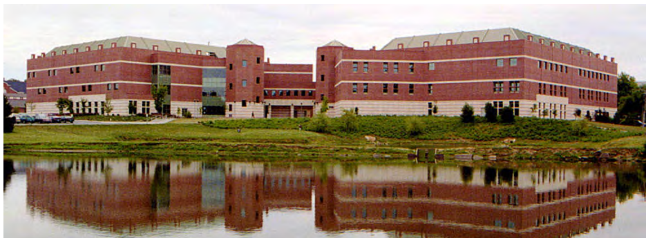
Victaulic's BIM services and Installation-Ready couplings saved EMC 30 percent in labor costs as they renovated Building 120 (Eisenhower Hall) at U.S. Army post Fort Leavenworth. Projects included replacing the existing HVAC system with a more energy-efficient hybrid geexchange system featuring 240 geothermal wells.
