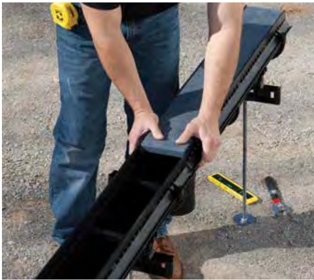
3. Ensure that channels are securely connected and properly seated in the Rante Arrow™ - Figure Number 9849NS.
