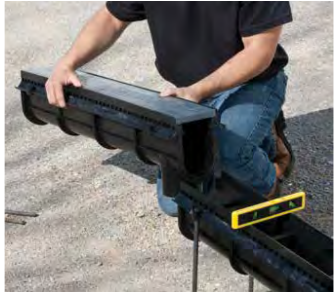
2. Align male and female ends of the channels.
