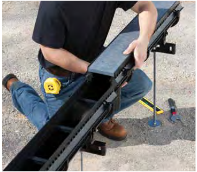
2. Slide channels together.
