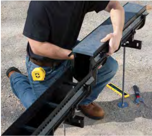
1. Align male and female ends of the channels.
