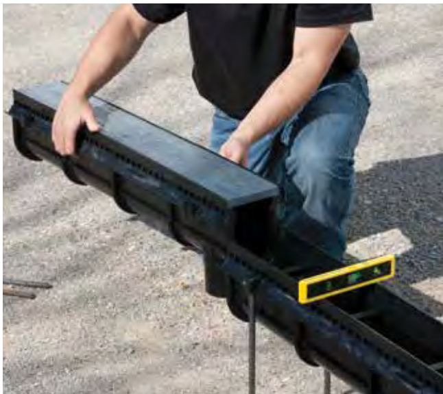
3. Slide channels together. Ensure that channels are securely connected and correctly aligned.
