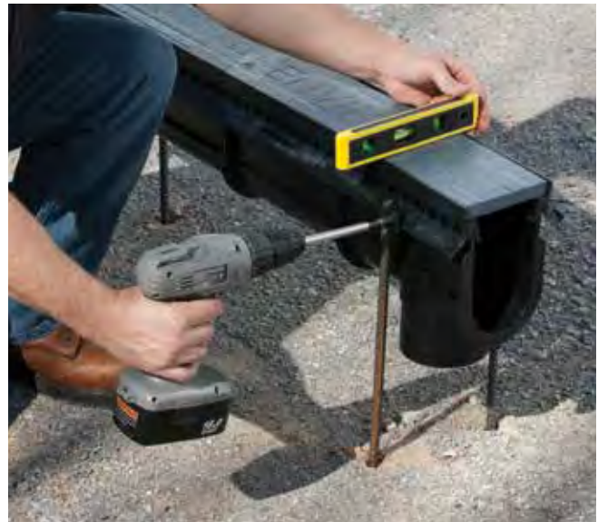
4. Secure channel into the ground with rebar using integral rebar clips.
